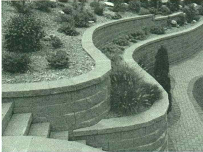
Illustration 1133.08(e)(5)(B): This image illustrates a retaining wall that has been benched so that there is not a single, excessively tall, retaining wall.
